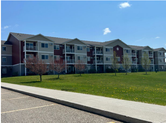
Sunset Ridge Apartments
